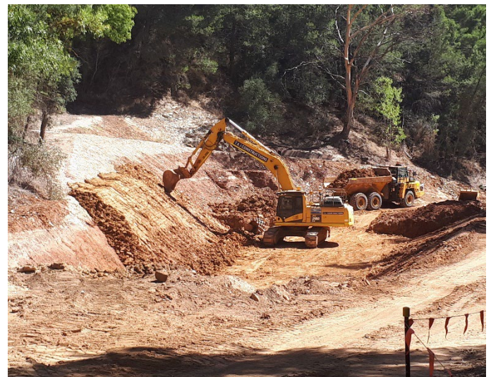
Image: SB2 under construction.
