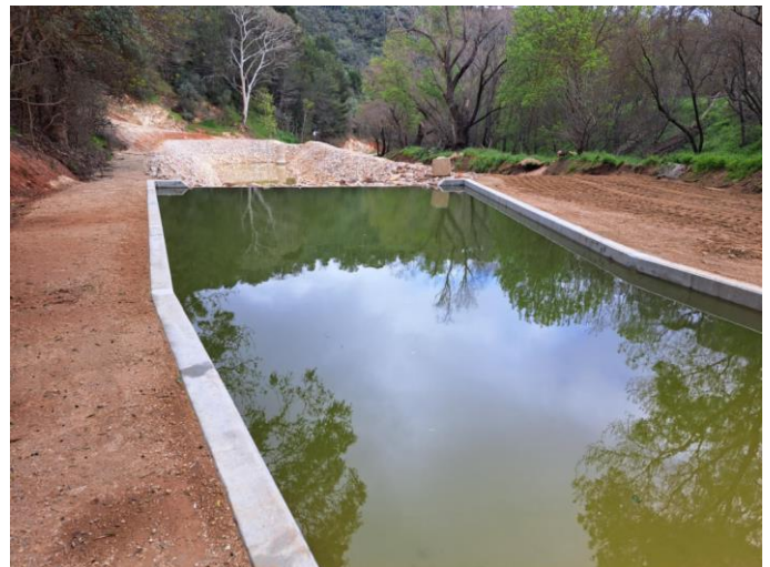
Image: New SB2A facing west – concrete forebay
