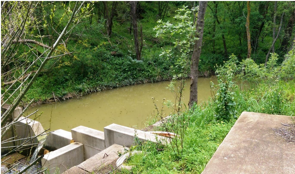
Figure 5-1 : Concrete Step Weir
