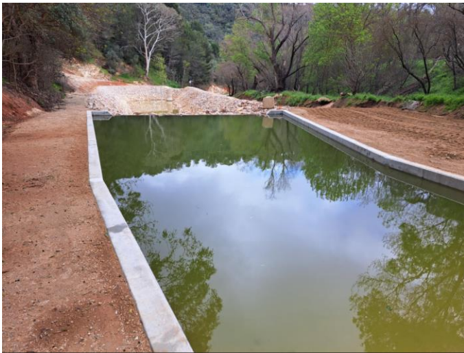
Image: New SB2A facing west – concrete forebay
