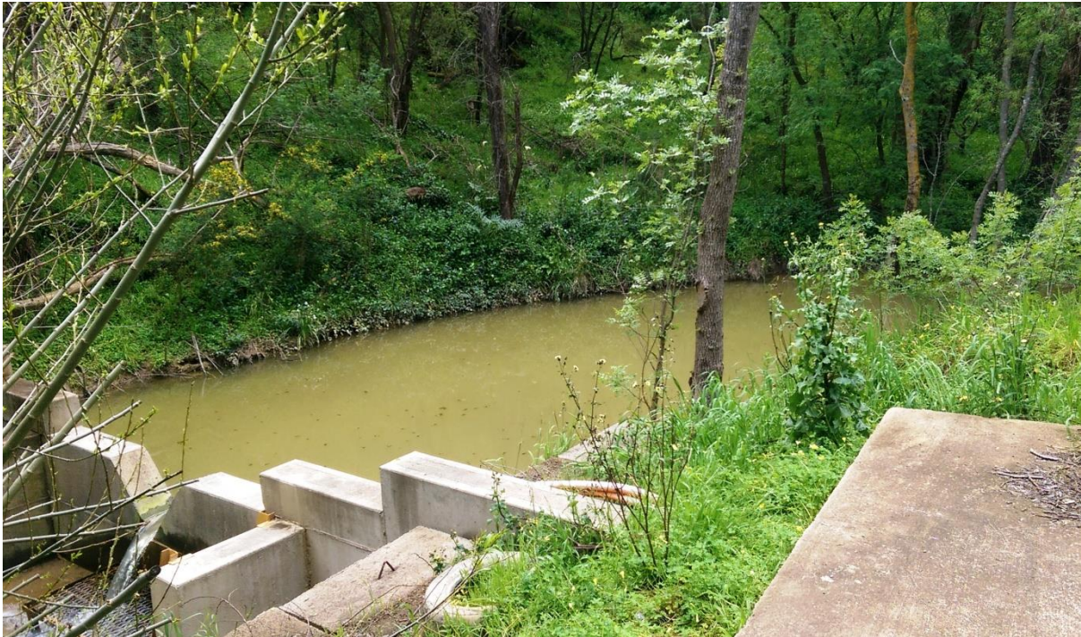
Figure 5-1 : Concrete Step Weir
