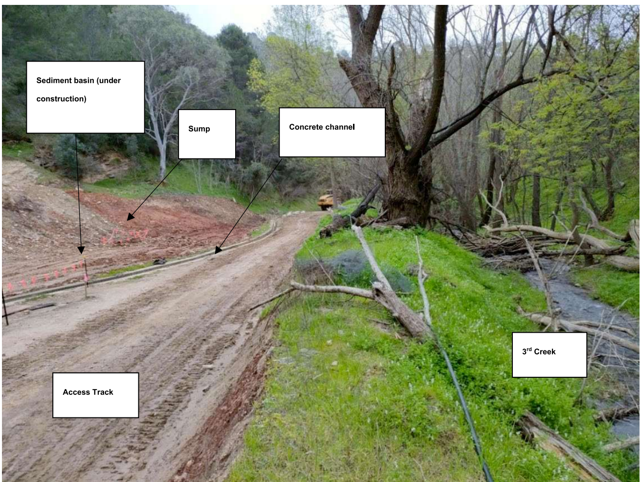
Figure 2. Location of detention basin with respect to 3 rd Creek and the Site access Road. Key features denoted.
