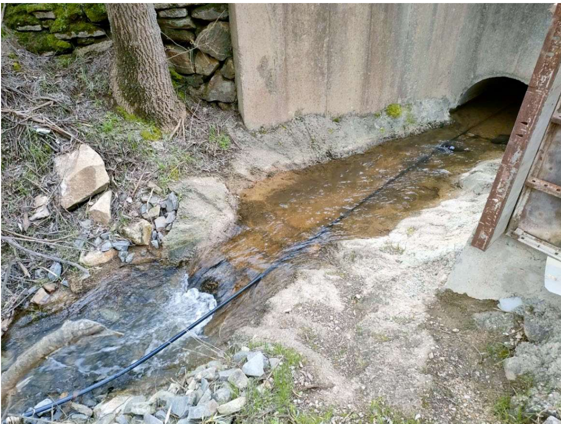
Figure 4. 3 rd Creek at the time of inspection.
