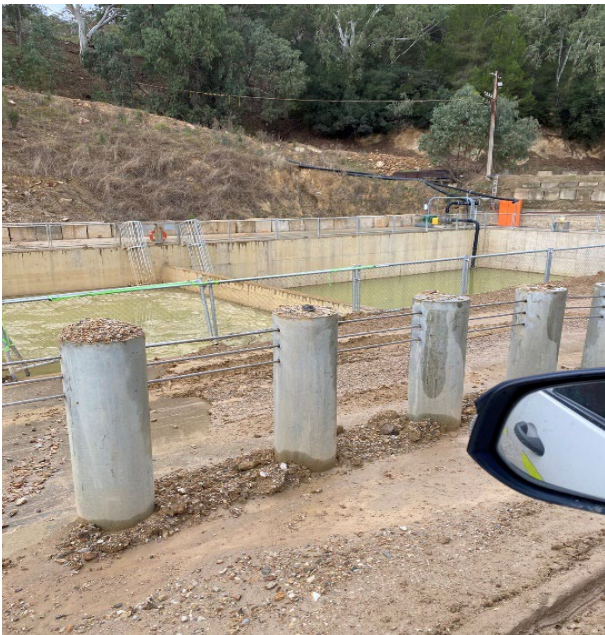
Photo 3.1: Main sediment collection system and source of stockpiled soil
