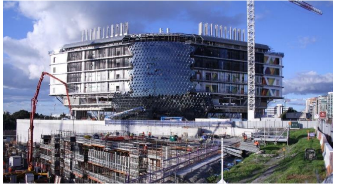
Image: SAHMRI under construction
