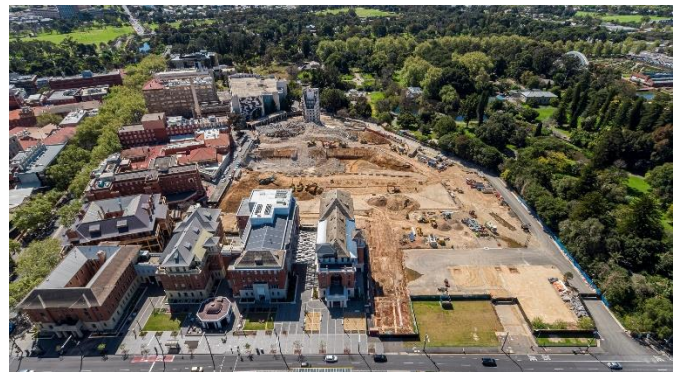
Image: Lot Fourteen under construction.
