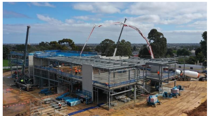
Image: Morialta Secondary College under construction.
