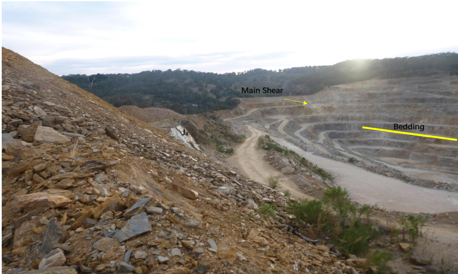
Plate 16: This image shows a few of the main structures on site which have been considered as part of the geotechnical assessment.
