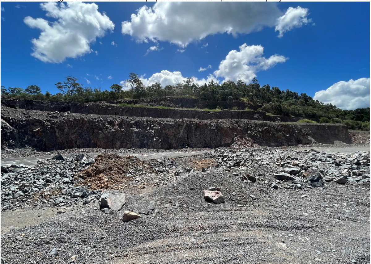
Plate 13: A view of the ongoing rehabilitation at another quarry with rehabilitation completed in the right and moving slowly to the left of page.
