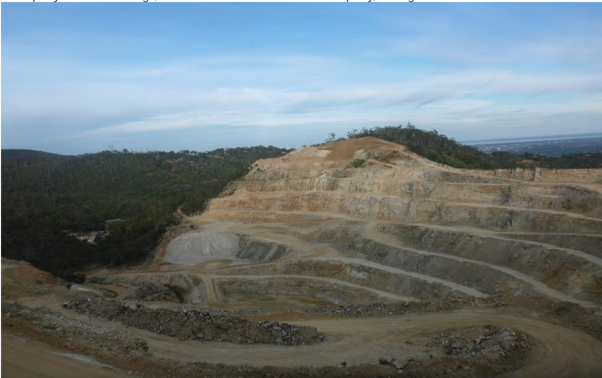
Plate 9: The west wall of White Rock Quarry is similarly already a very significant slope which shows no material signs or vectors denoting slope instability.
