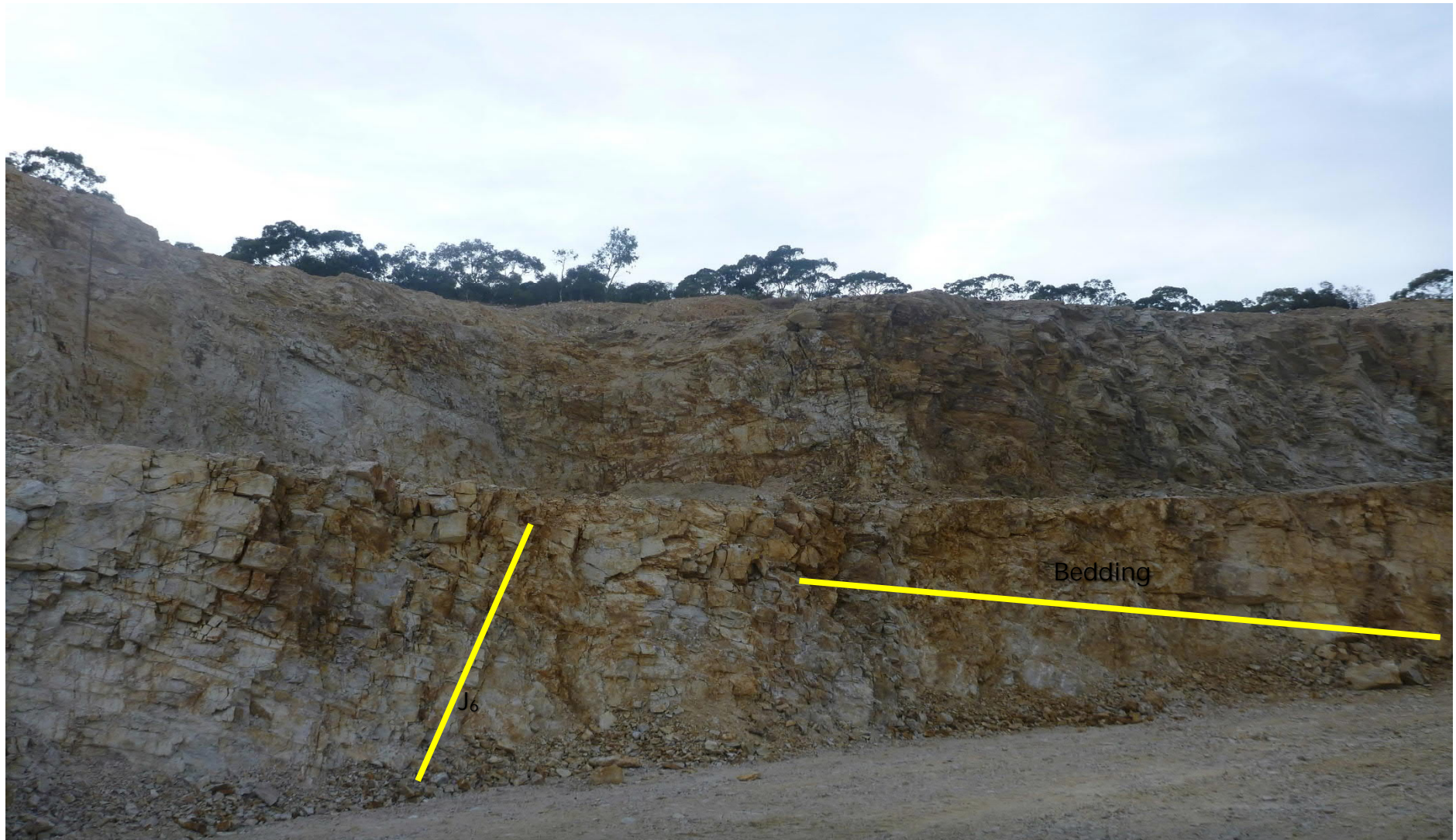
Plate 17: A further image which shows the comparatively small block size the intensity of the jointing and the degree of weathering encountered on site in the upper benches.
