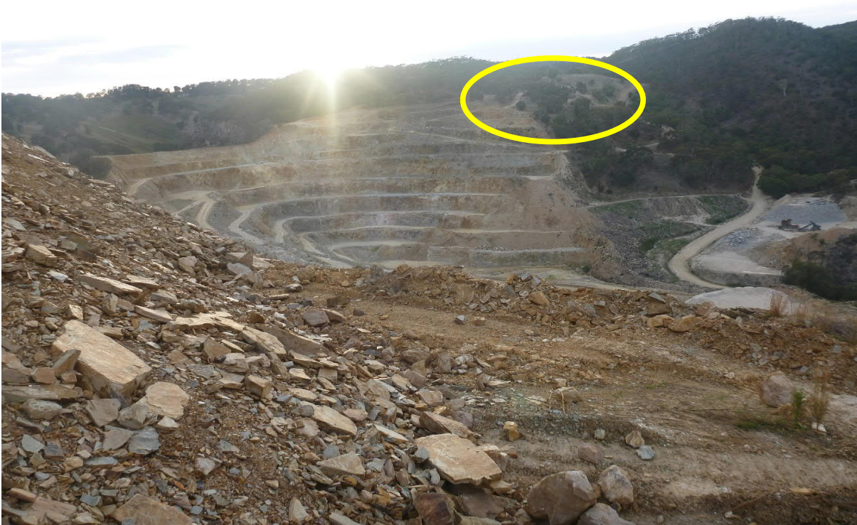
Plate 8: The White Rock Quarry is already a significant operation which has a current total slope height of 120 metres in the east wall which will not materially change resultant of this proposal in the final bench heights. That is the slope heights which currently exist will not significantly change and the driving and gravitational forces which are currently managed by the slope design are expected to be similarly managed by the future design which largely uses the same design criteria. The overburden (yellow circle) is also partly visible in this image, which is treated as an extension of the quarry, although several areas of overburden exist.
